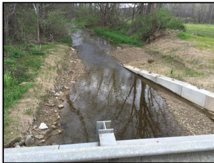
Image 2: Example single arm rock vane installation using precast concrete bin blocks.
