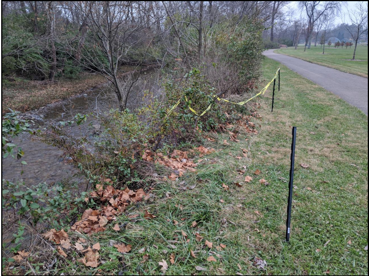
Image 4: Existing streambank erosion near Senior Center.
