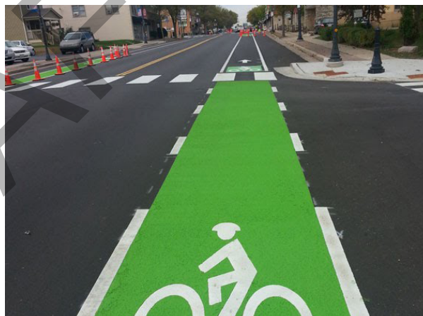
Green painted lanes are an effective way to draw attention to cyclists, particularly at intersections.
