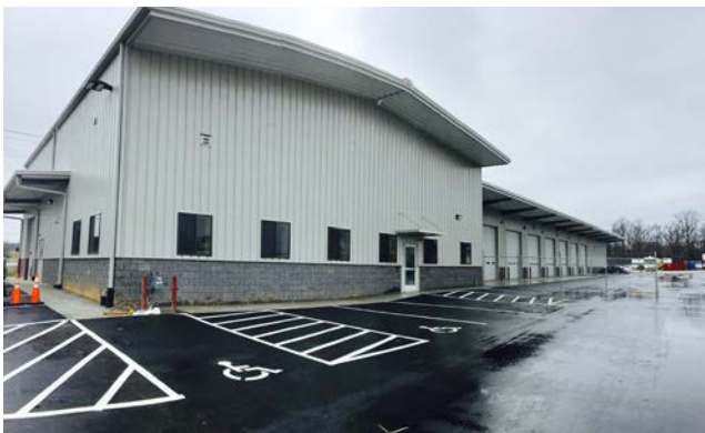
Image: Warehouse Building
