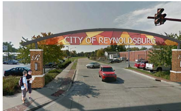
Main Street and Davidson Drive (looking south).
