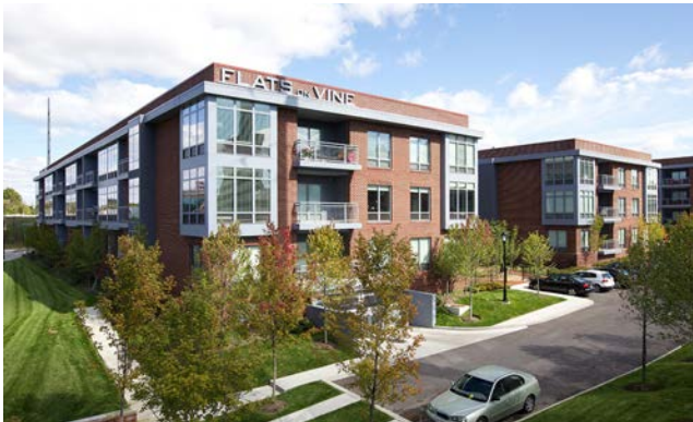
Image: Multi-Unit Building
