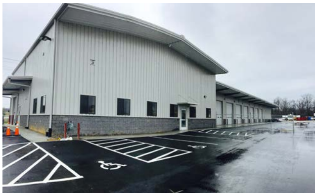
Image: Warehouse Building
