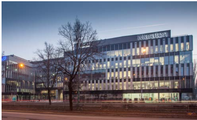
Image: Office-Corporate Building
