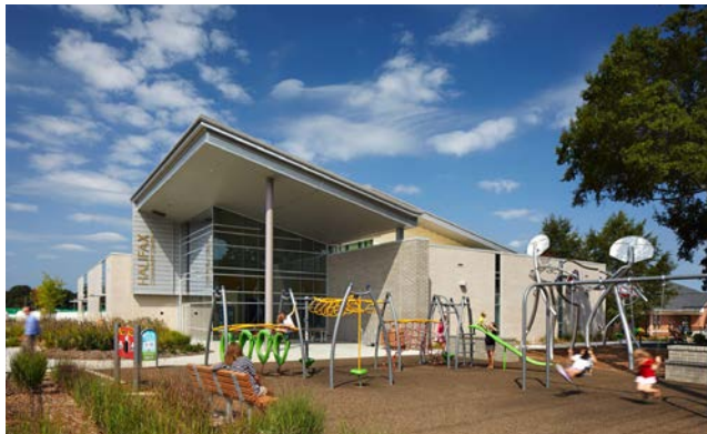
Image: Community Activity Center Building
