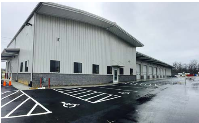
Image: Warehouse Building
