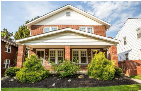
Image: Duplex Building
