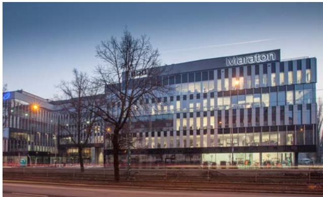
Image: Office-Corporate Building
