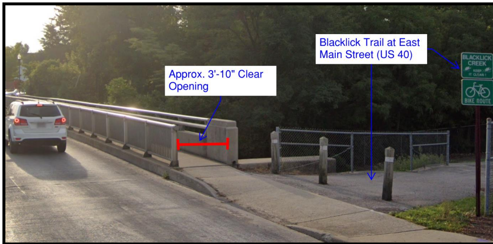
Figure 3: Blacklick Trail at East Main Street Bridge Crossing
