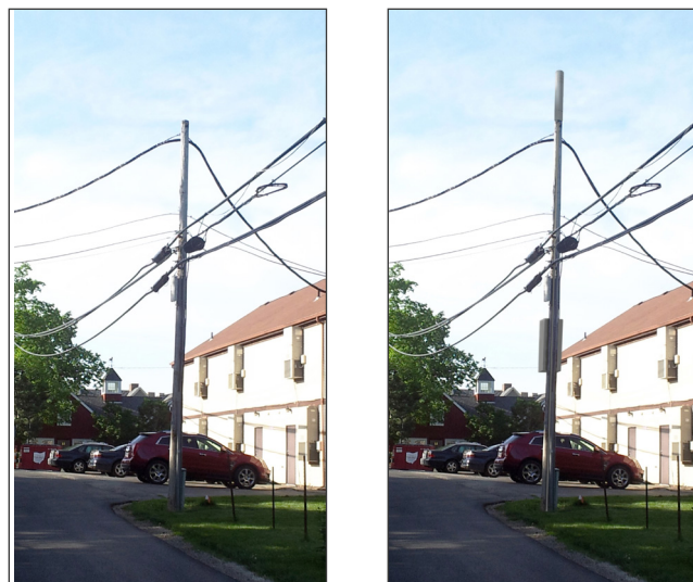
Figure 5.1B--Illustrative Type 1 Collocation Request on Existing Private Wooden Utility Pole (at right)
