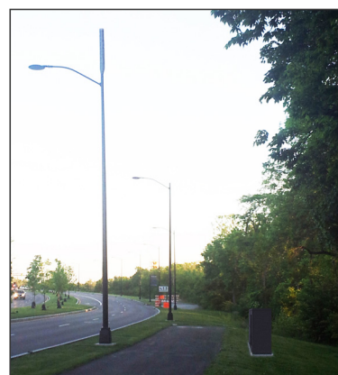
Figure 5.2C--Illustration of Type 1 Collocation with Ground-mounted Small Cell Equipment along Open Space within the Right-of-Way.
