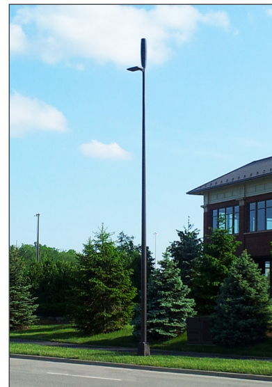
Figure 5.5A--Illustration of Collocation on Existing Standard Light Pole with Ground-mounted Facilities Cabinet Integrated into Existing Landscaping
