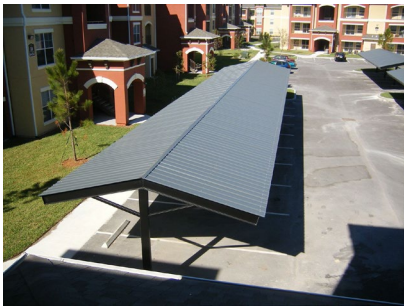
Example of canopy/carport
