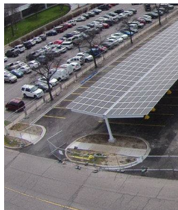
Example of canopy/carport with solar panels
