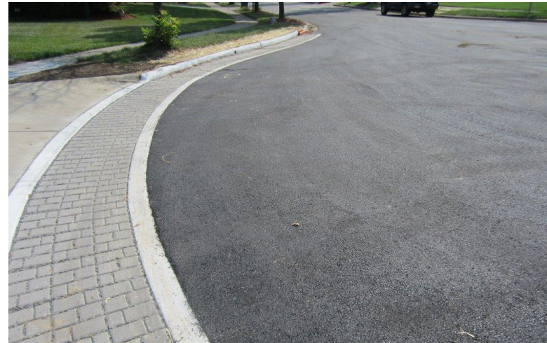
Cul de sac stormwater storage retrofit
