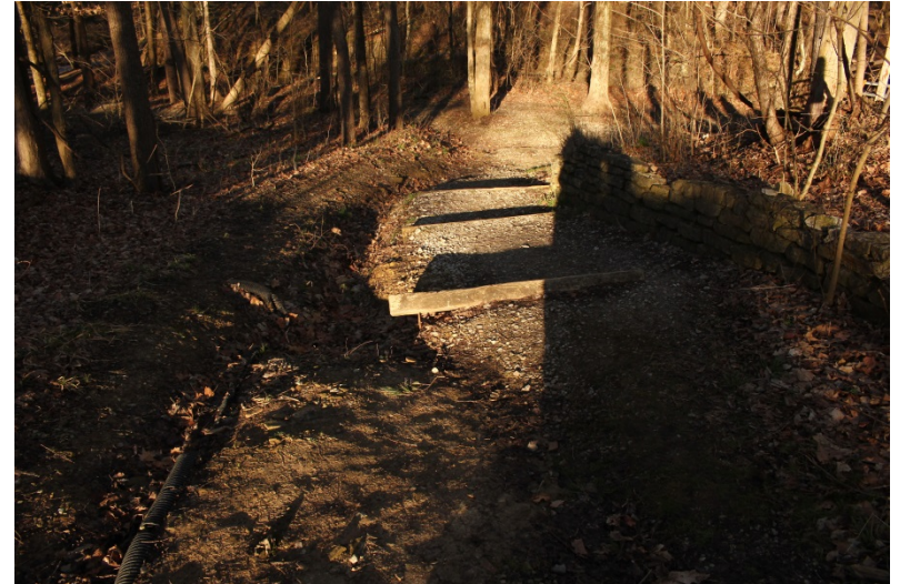
Erosion in Pine Quarry Park from a single rain event
