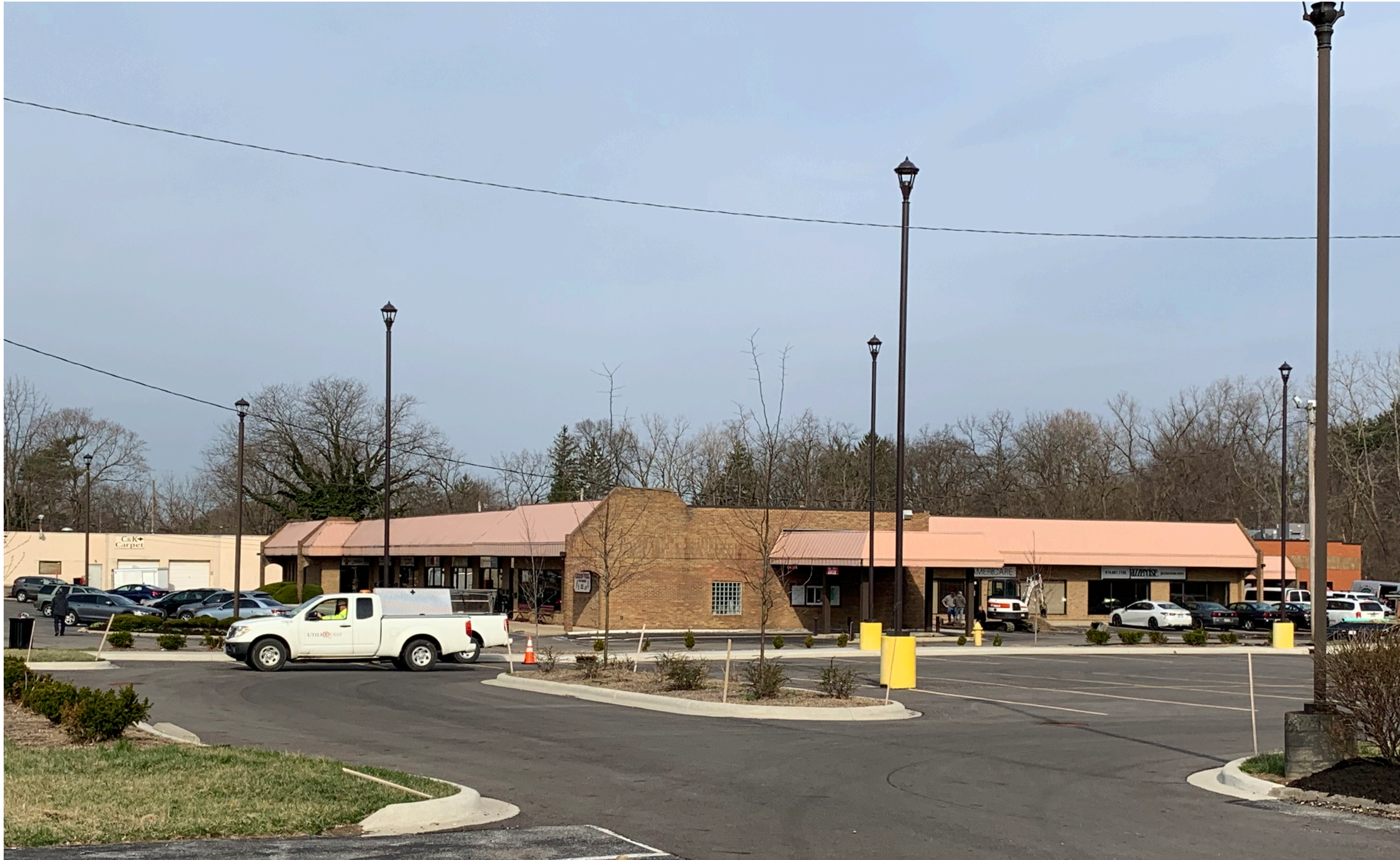
EXISTING WEST BUILDING
