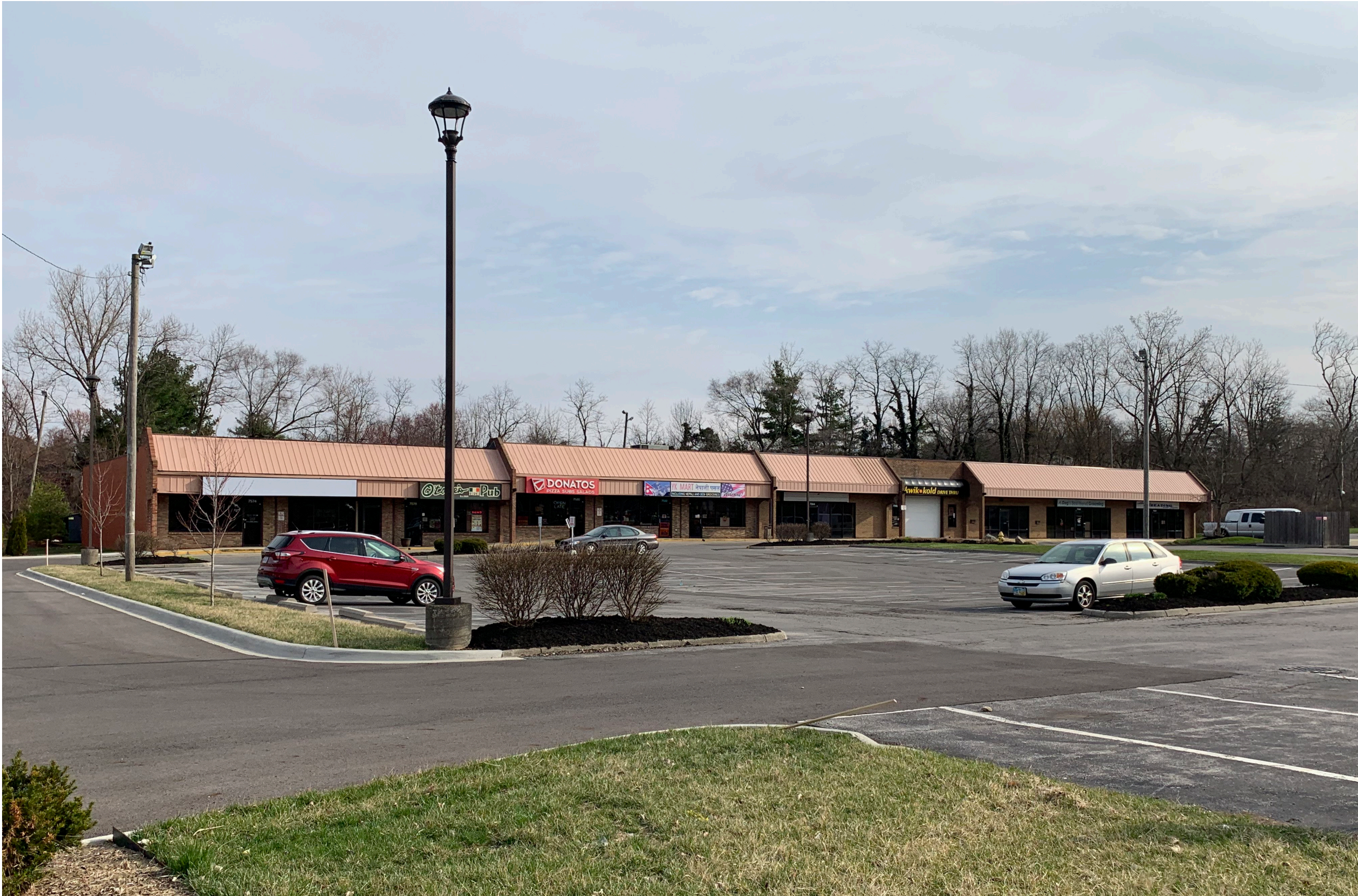
EXISTING EAST BUILDING
