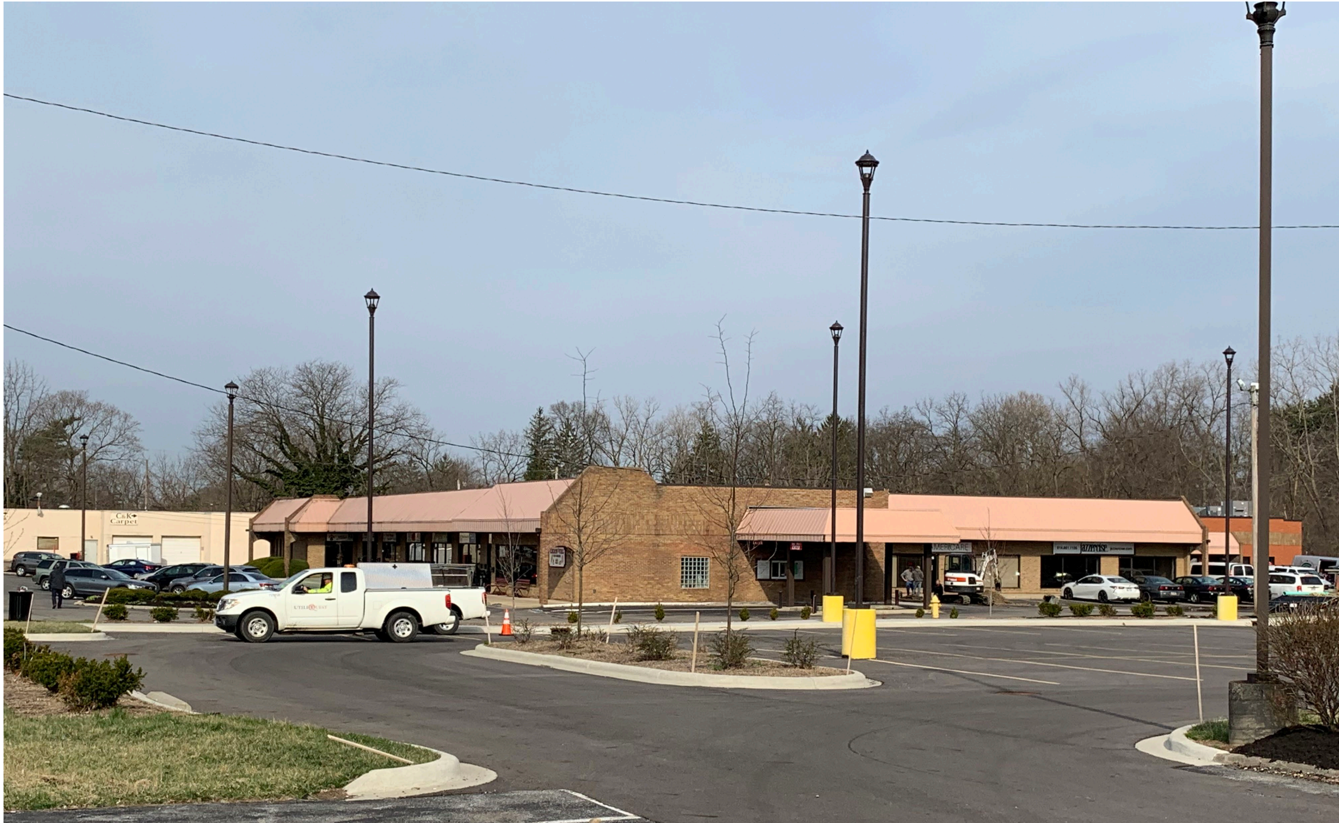
EXISTING WEST BUILDING
