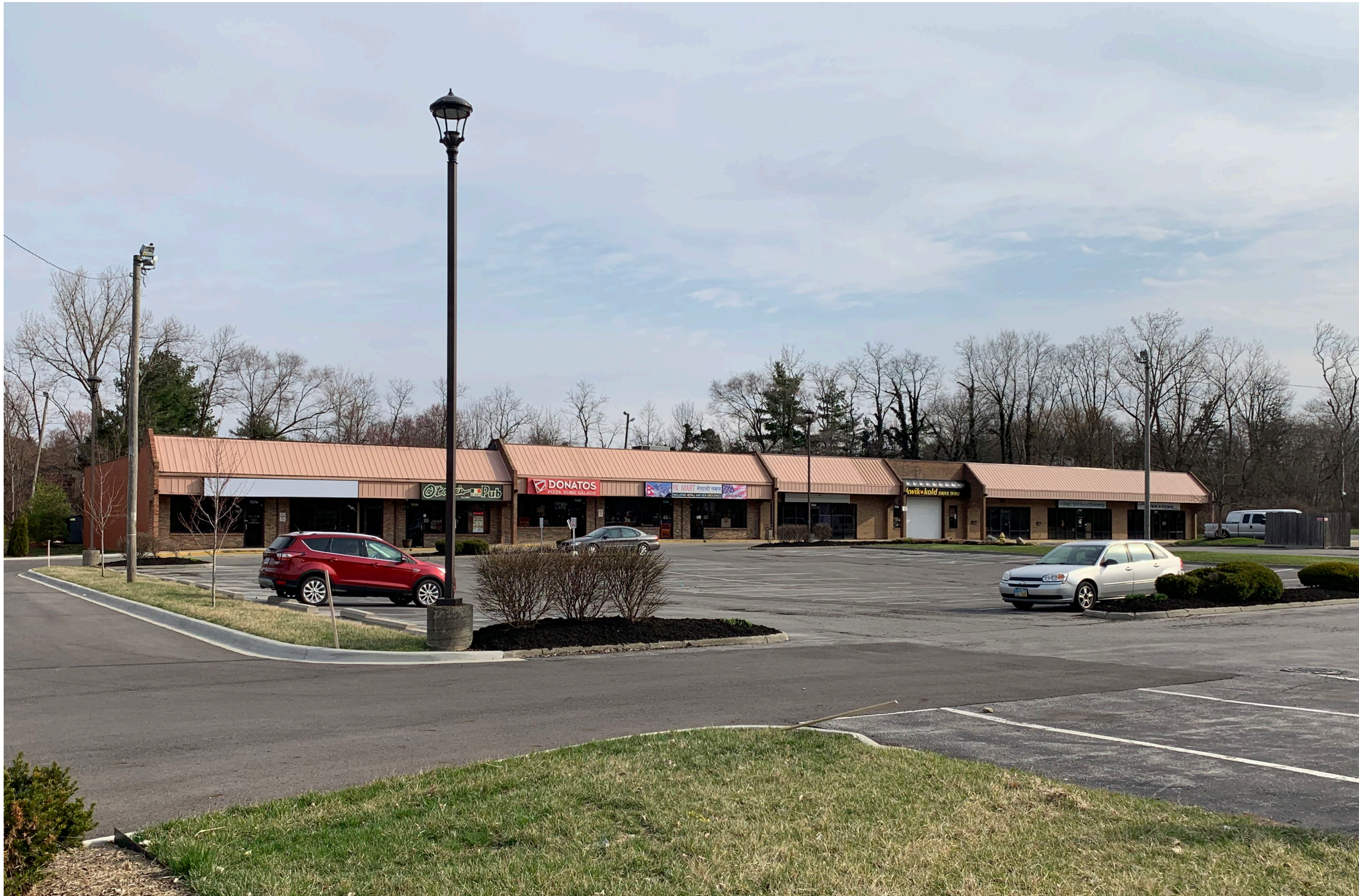
EXISTING EAST BUILDING
