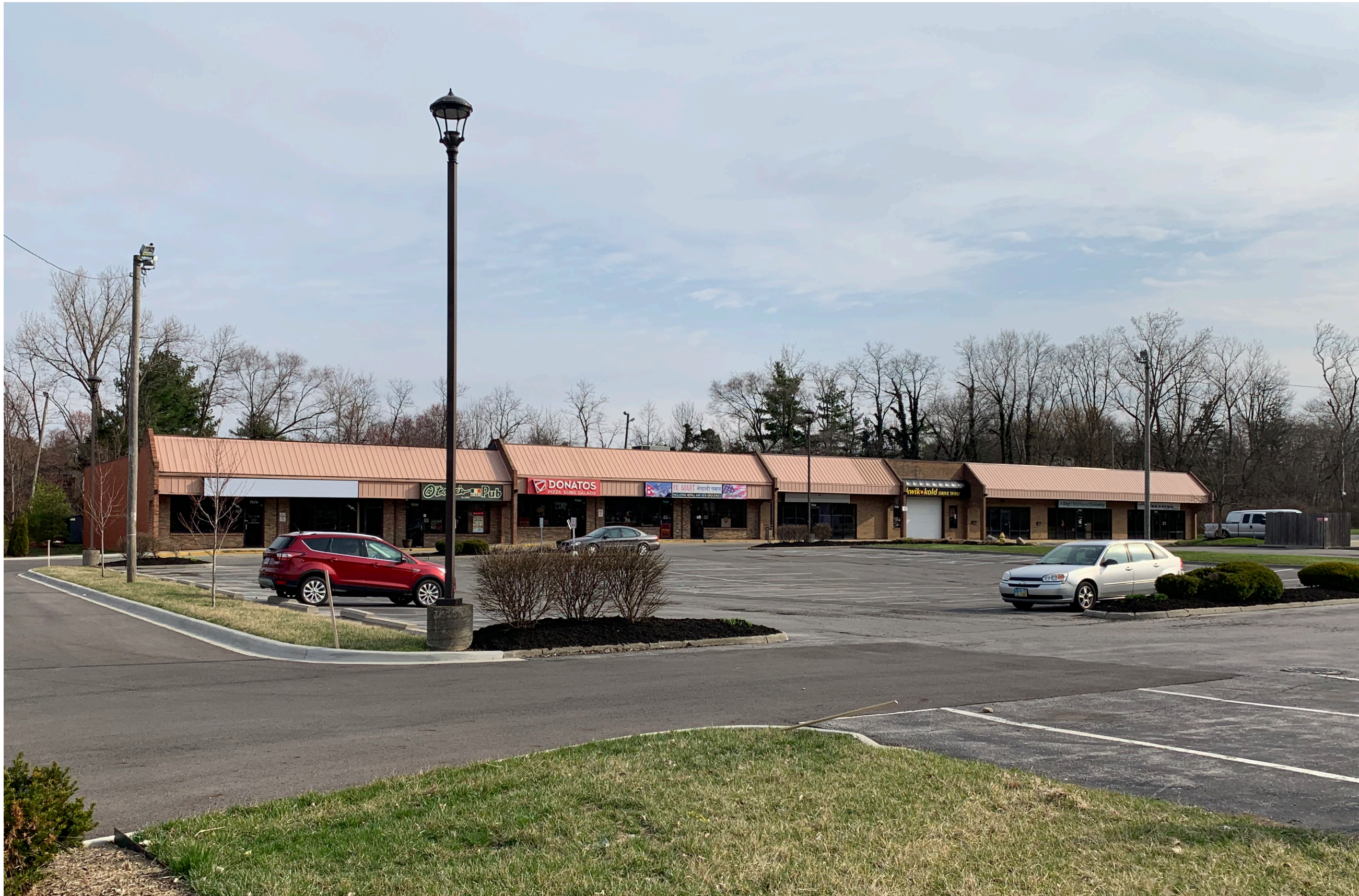
EXISTING EAST BUILDING
