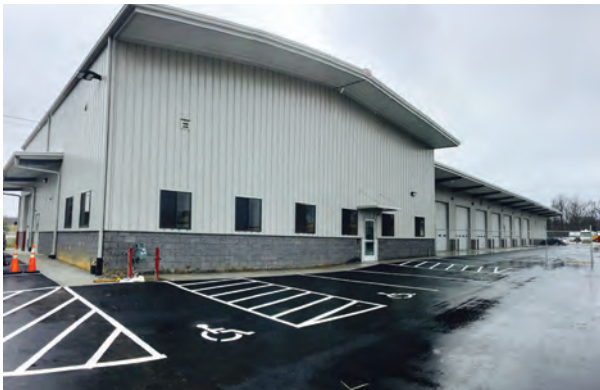
Image: Warehouse Building
