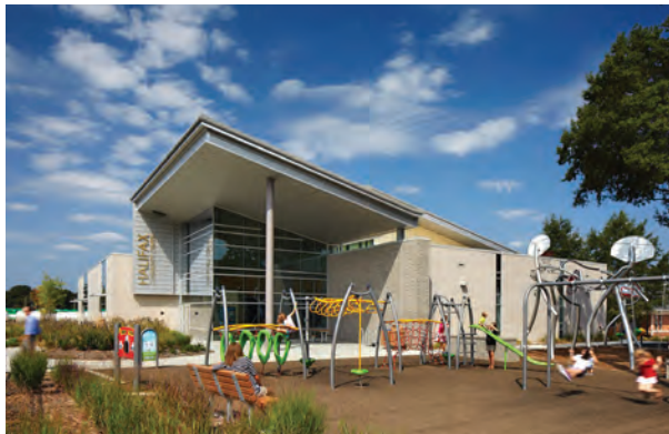
Image: Community Activity Center Building
