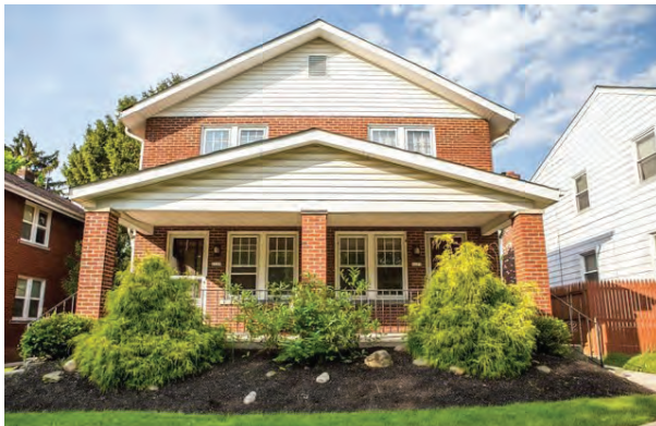
Image: Duplex Building
