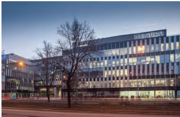
Image: Office-Corporate Building
