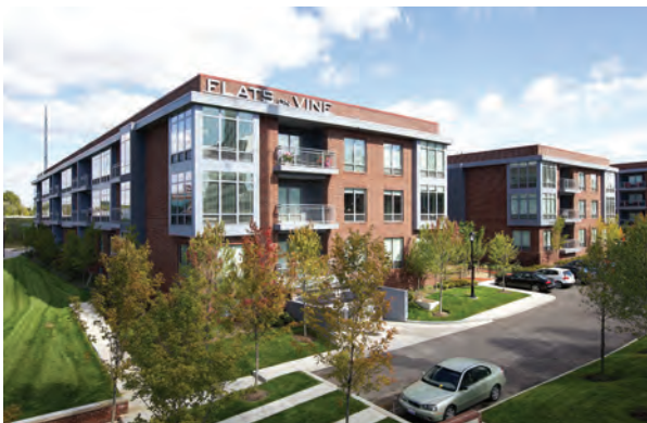
Image: Multi-Unit Building
