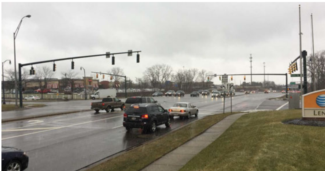
State Route 256 looking toward the Taylor Road
