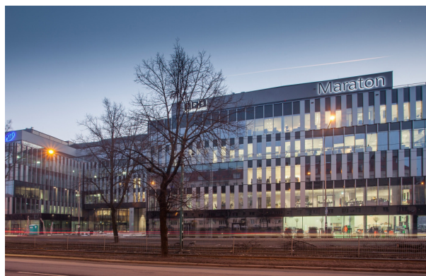
Image: Office-Corporate Building
