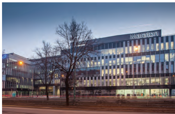
Image: Office-Corporate Building
