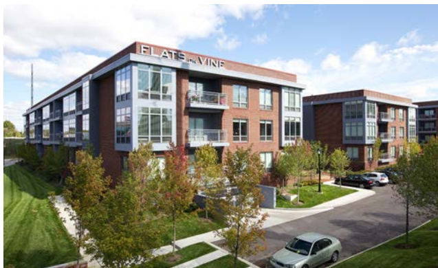
Image: Multi-Unit Building
