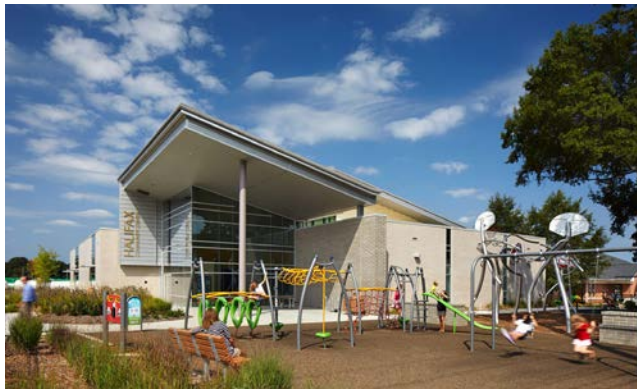
Image: Community Activity Center Building
