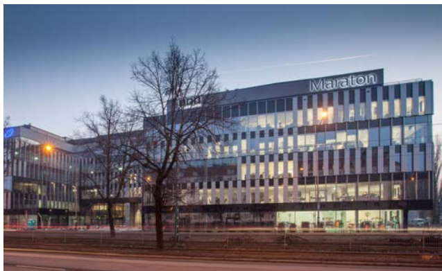
Image: Office-Corporate Building
