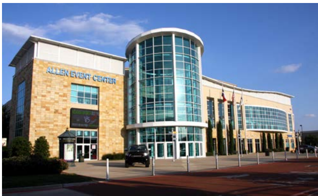
Image: Event Center Building
