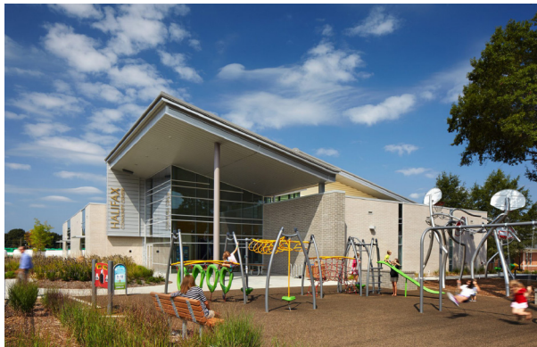
Image: Community Activity Center Building
