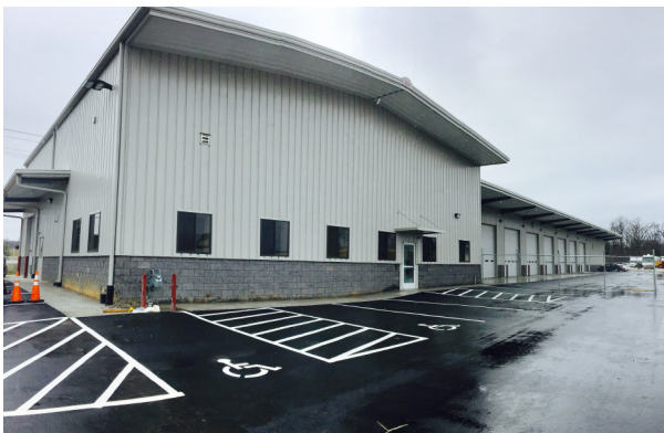
Image: Warehouse Building
