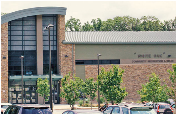
Image: Community Center Building
