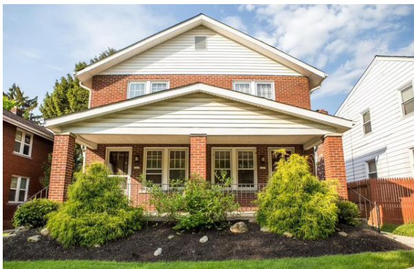
Image: Duplex Building
