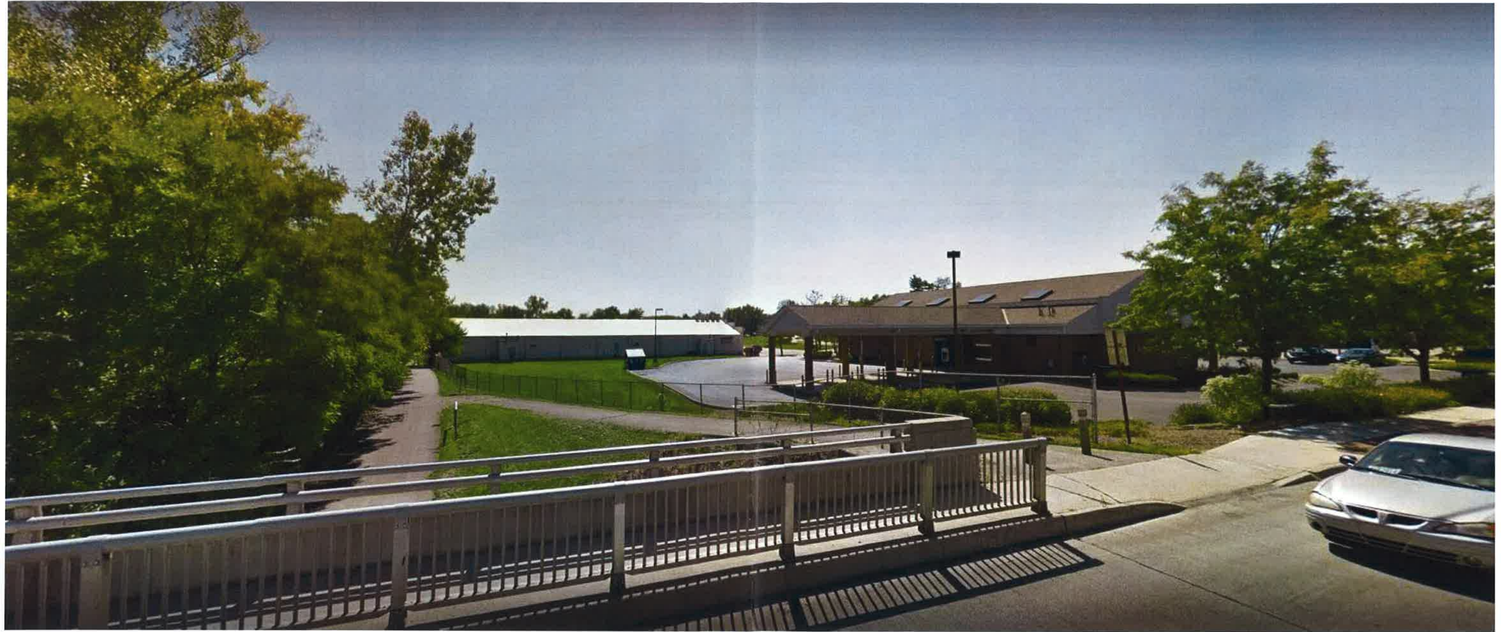
OVERALL STREET VIEW - SIDE
