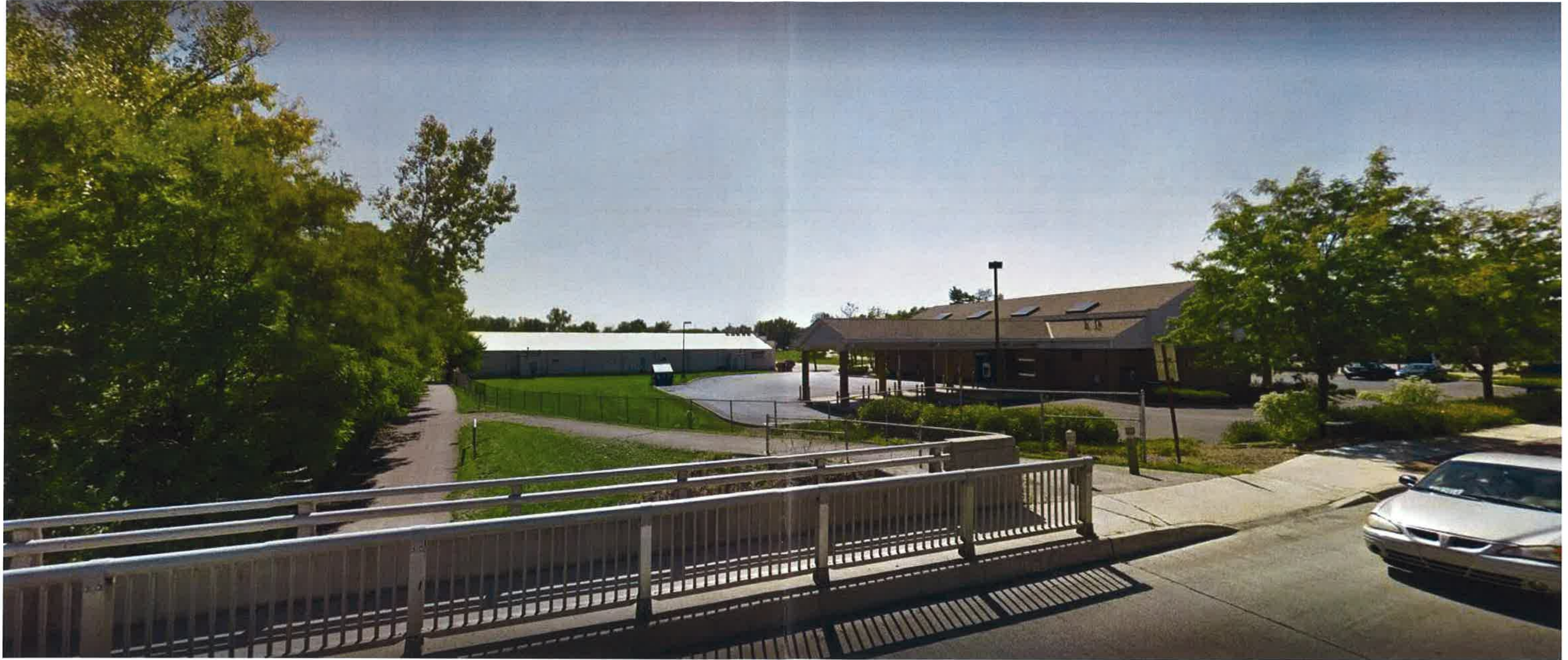
OVERALL STREET VIEW - SIDE
