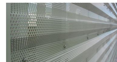
MECHANCIAL SCREEN (MTL-4): PERFORATED ANODIZED ALUMINUM
