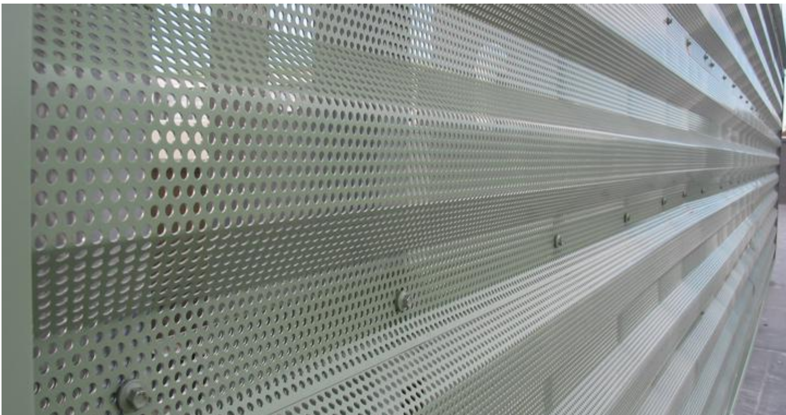
MECHANCIAL SCREEN (MTL-4): PERFORATED ANODIZED ALUMINUM
