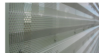
MECHANICAL SCREEN (MTL-4): PERFORATED ANODIZED ALUMINUM
