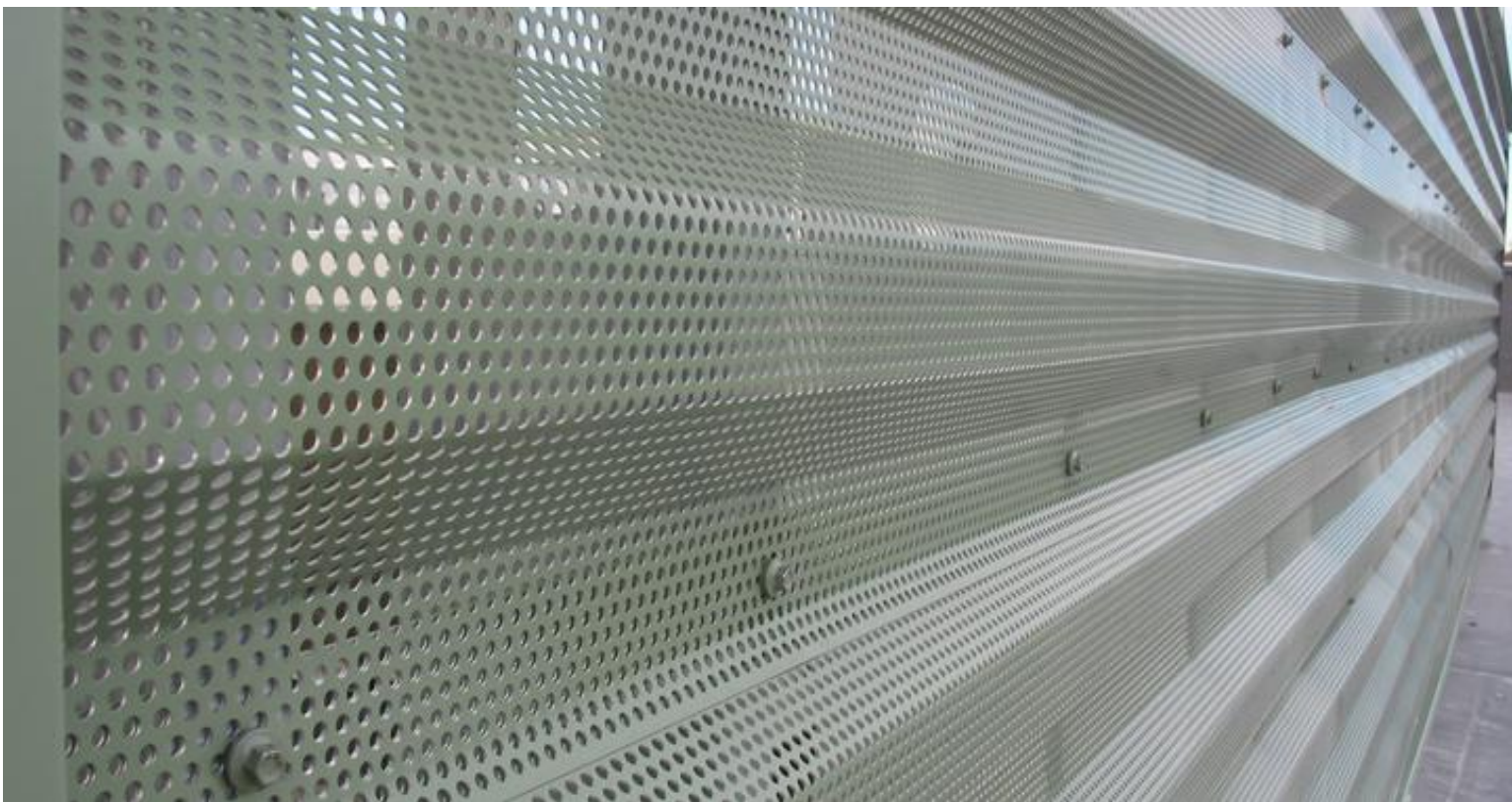
MECHANCIAL SCREEN (MTL-4): PERFORATED ANODIZED ALUMINUM
