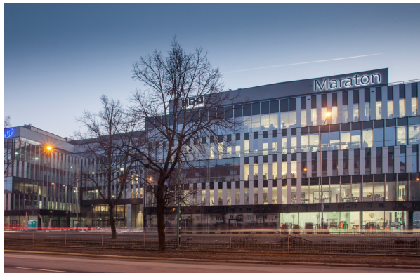
Image: Office-Corporate Building
