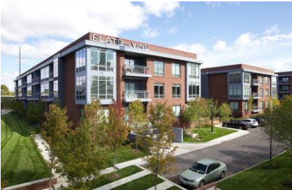
Image: Multi-Unit Building
