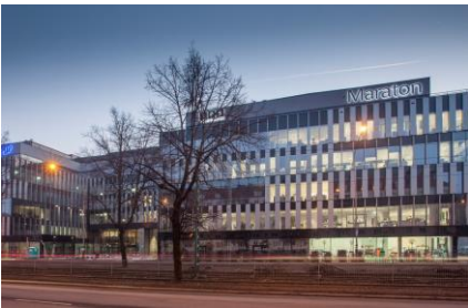
Image: Office-Corporate Building
