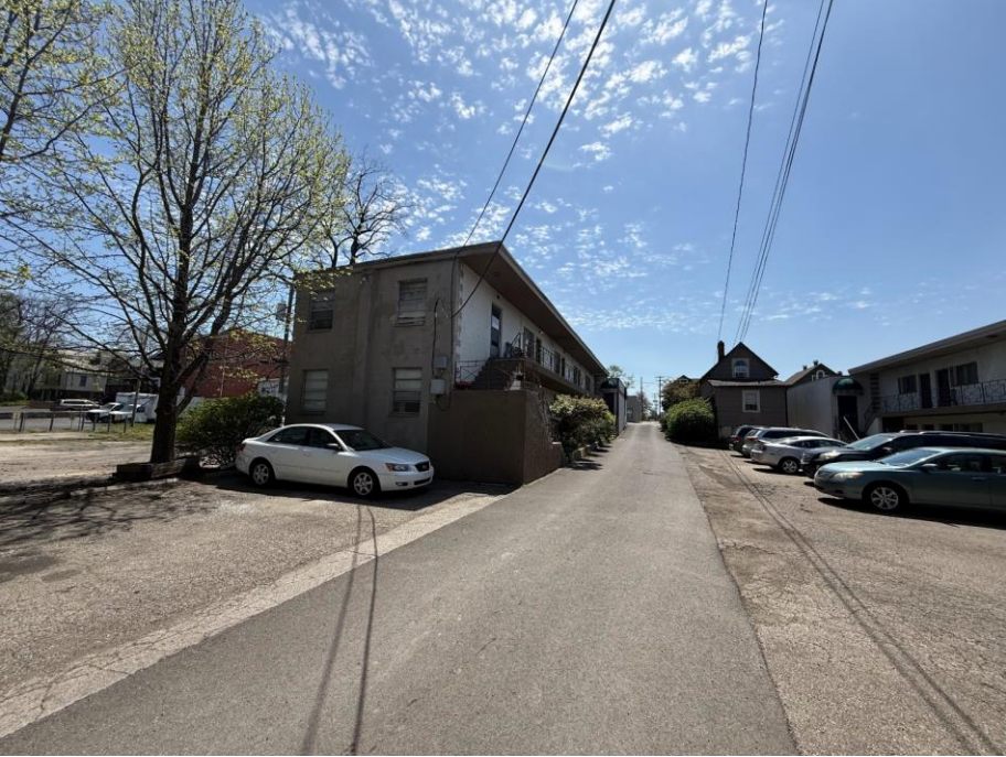
This is a view from the back of the property looking toward E Main St. The back wall has 4 windows that will be replaced and we will be painting that entire side of the building.
