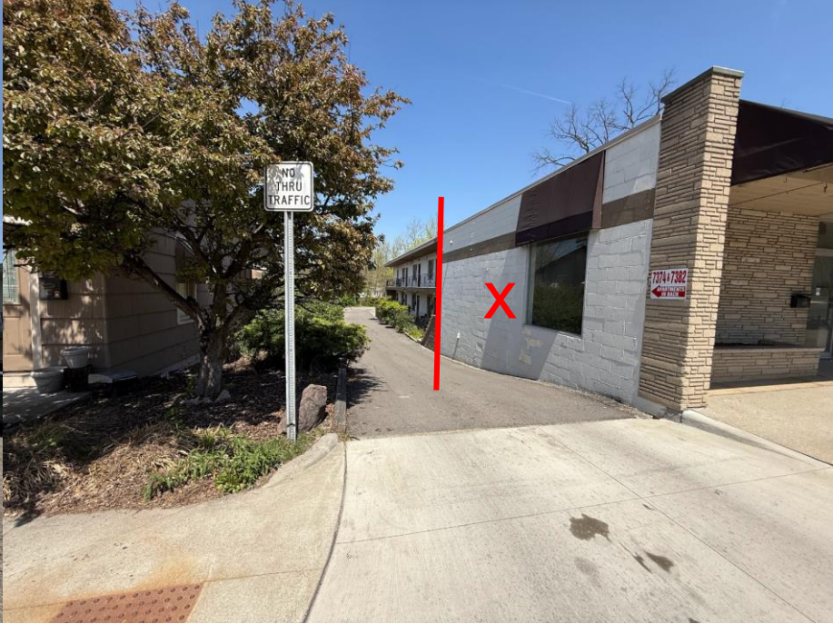
This is a view of the property from E Main Street. The storefront (marked with a red X) will not be touched. Left of the red line is the 10 residential units that will receive new windows, doors and paint.
