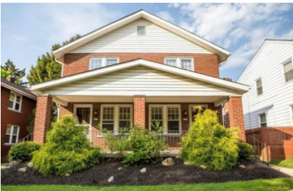
Image: Duplex Building
