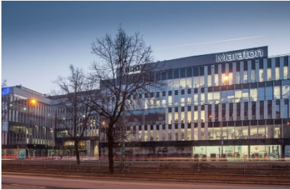
Image: Office-Corporate Building
