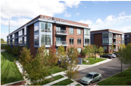
Image: Multi-Unit Building
