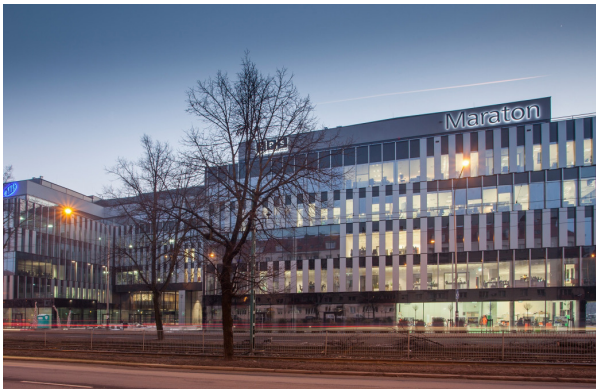
Image: Office-Corporate Building
