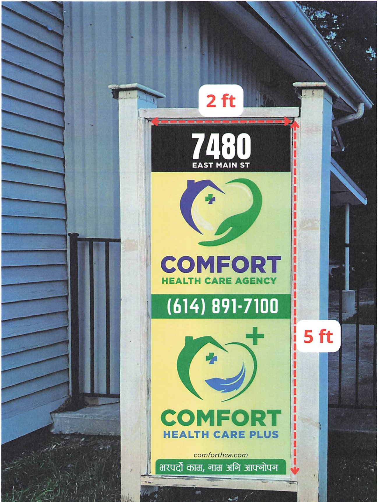
Refacing an old double sided business sign by replacing the face and graphics, while keeping the existing structure.
