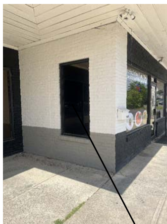
New Door Location to utilize existing window opening & header
